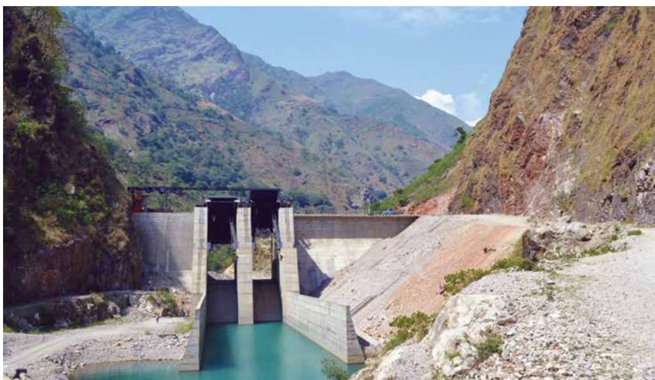
Photo 5.4: Chameliya hydropower project generates 30 MW electricity (Credit: Pradyumna Rana)
